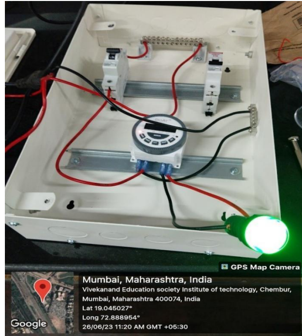
Figure 1: Control panel with automatic and manual modes
